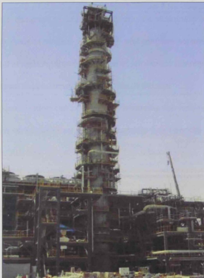
Figure 16: Condensate Stabilizer
