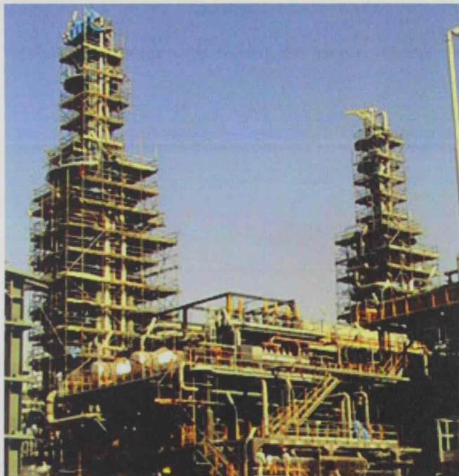
Figure 18: Condensate stabilizer columns under construction
