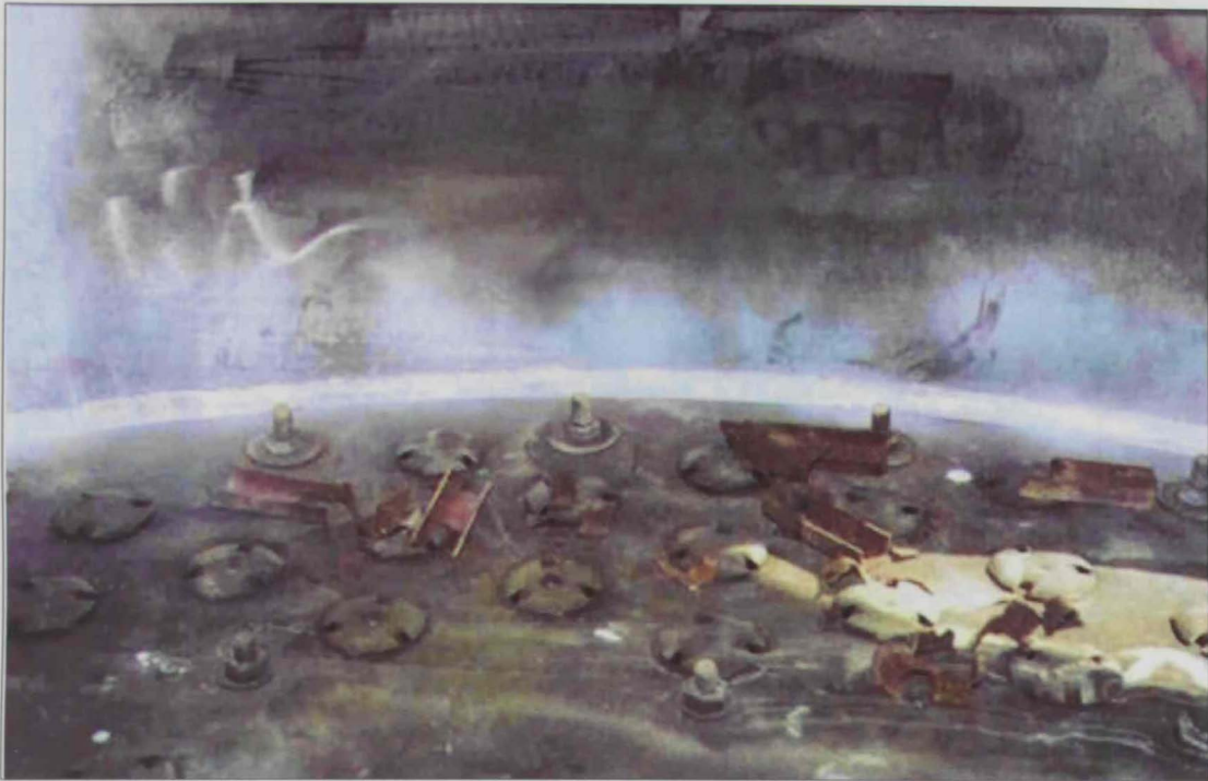
Figure 10: Broken clips which fell from upper trays due to cracking
